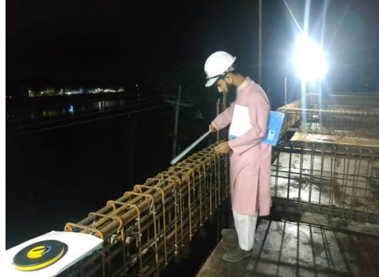
Cross check of rebar works 15 May 2026
