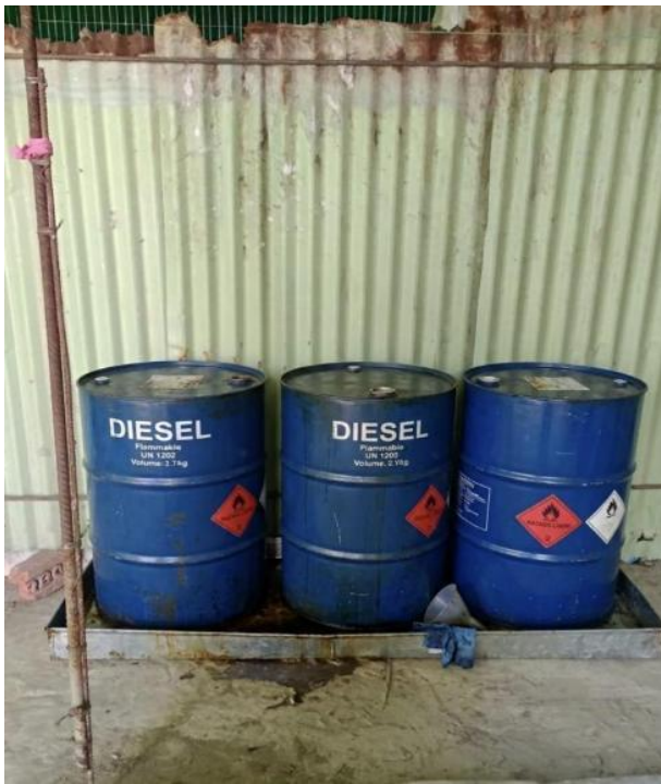
Fuel Storage with secondary containment, 03 June 2026
