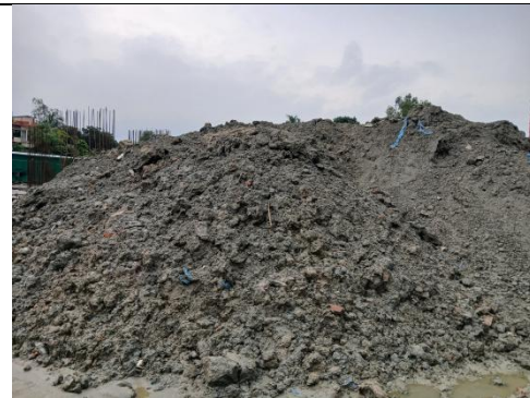
Temporary storage of excavated soil
