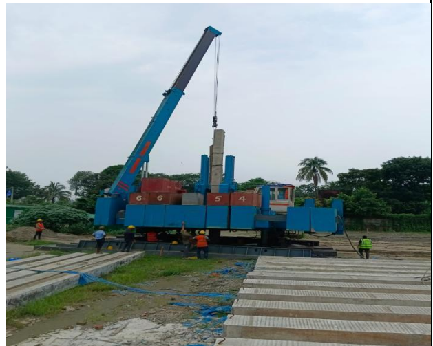
Pile Drive work, 27 June 2026
