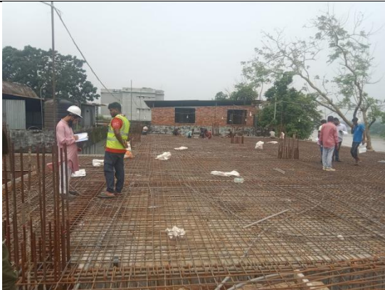
Rebar binding check 20 May 2026
