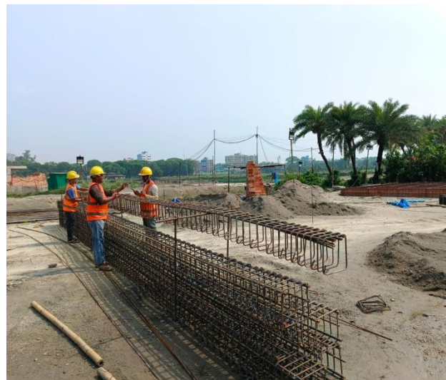
Rod Binding Work, 08 April 2026
