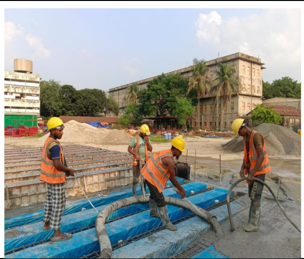
Pile Casting work, 05 March 2026
