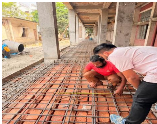
Cross check of rebar works
