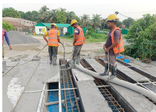
Pile Casting work, 13 May 2026
