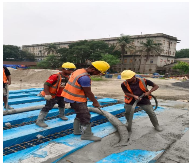
Pile Casting work, 11 April 2026
