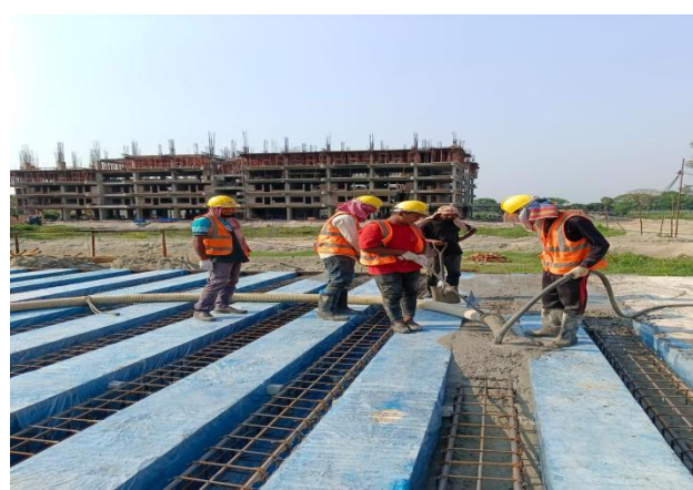
Pile Casting work, 16 May 2026
