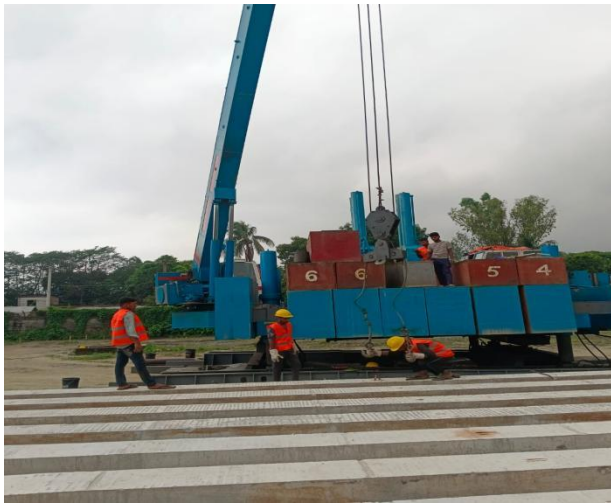
Pile Drive work, 24 June 2026
