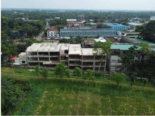
Aerial view of under construction building dated 26 June 2026
