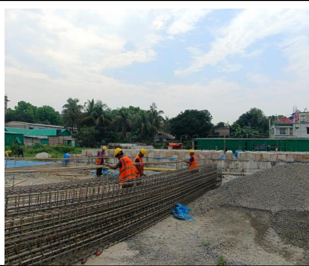
Rod Binding Work, 03 March 2026
