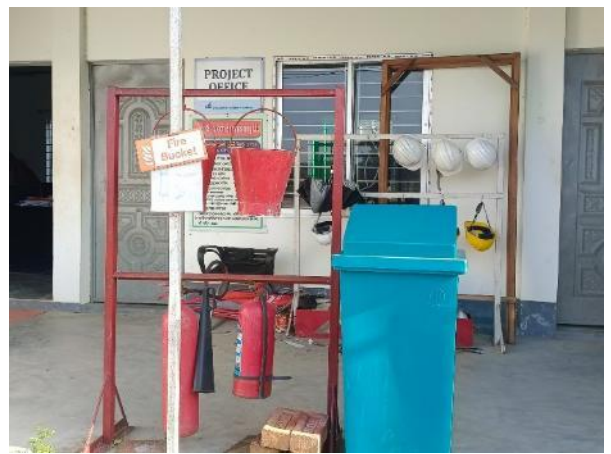
Fire extinguisher pressure check photo, 11 February 2026
