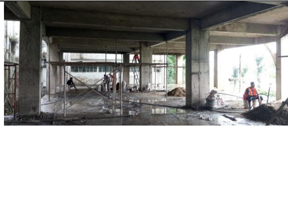
2 nd floor scaffolding removal works 24 June 2026
