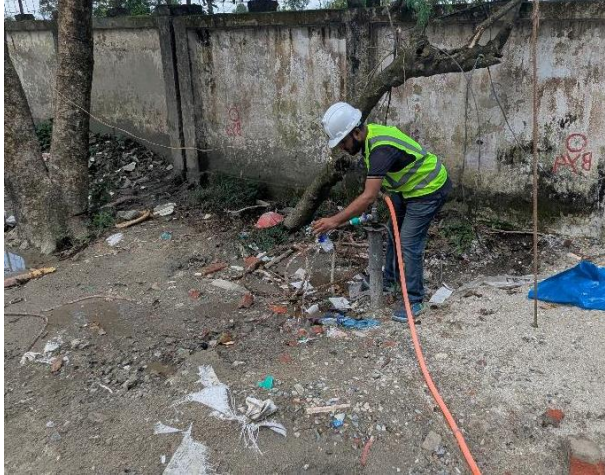
Photo (c1): Groundwater Sampling, GW-1, inside Project Site, Sylhet TTC
