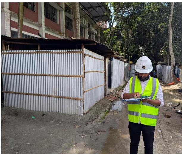
Photo (c2): NL2, Sylhet TTC Project Site
