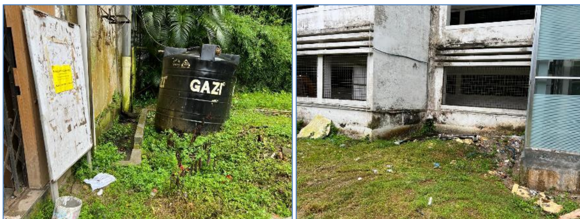
Figure VI-7 Images of the current drainage system at the proposed IBA site.
