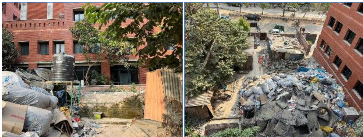
Figure 1: Proposed construction site for EDC EWU building
