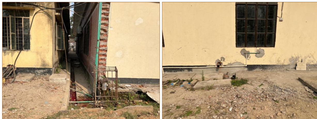
Figure III-4 Drainage system is functioning within the BUTEX campus.
