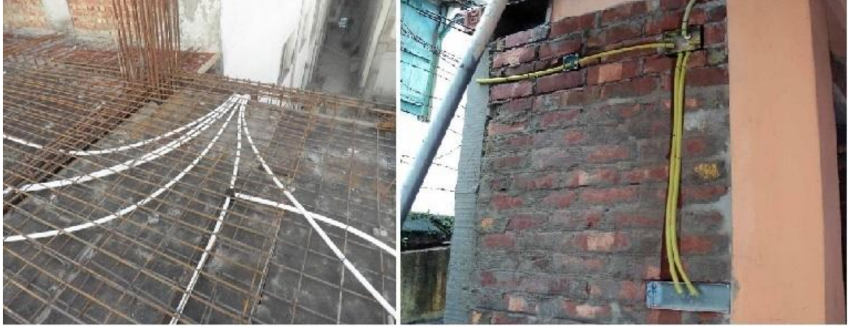
Concealed Conduit Installation in Slabs and Walls
