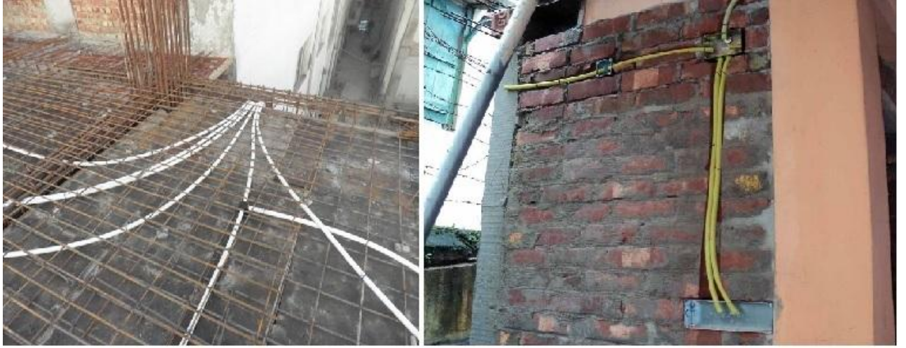
Concealed Conduit Installation in Slabs and Walls
