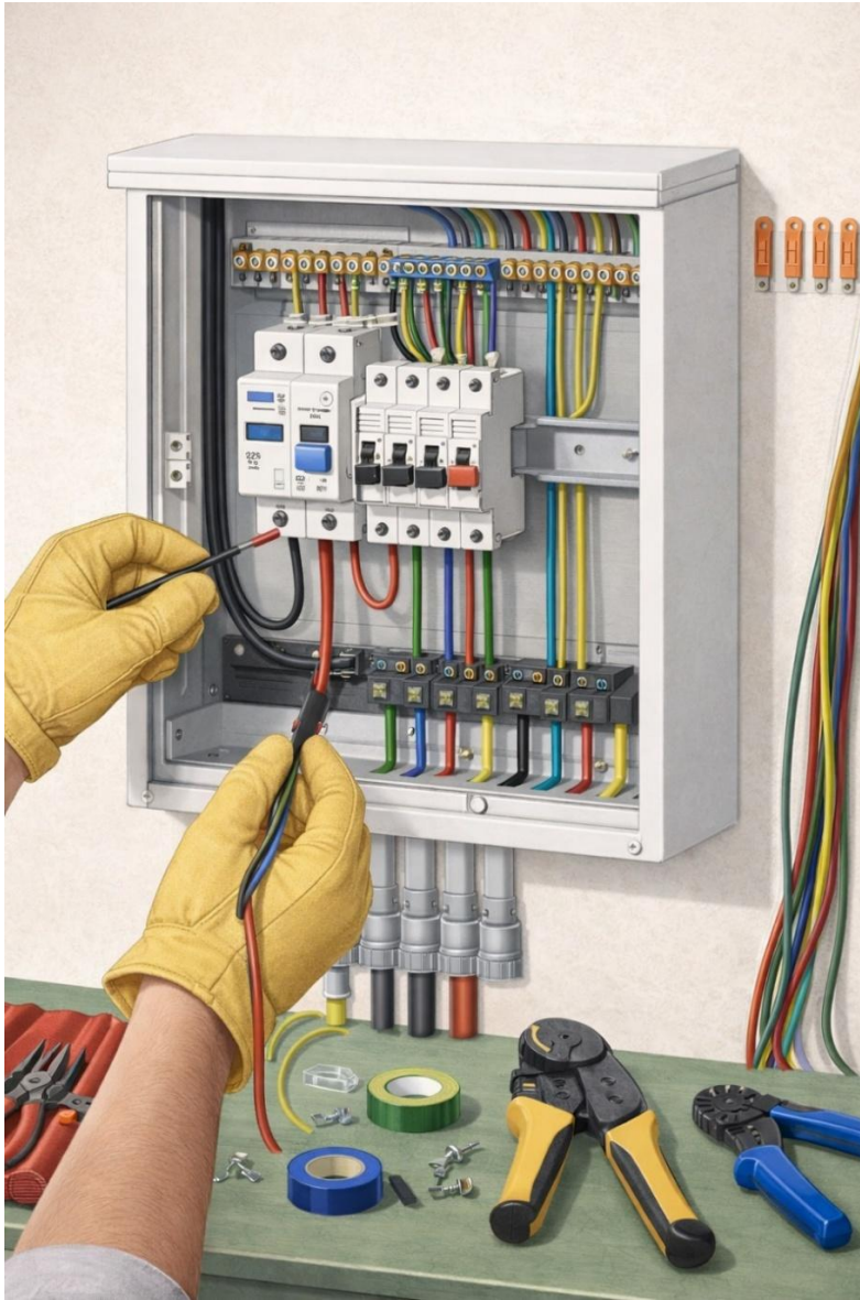
Installation & dressing of electrical distribution board
