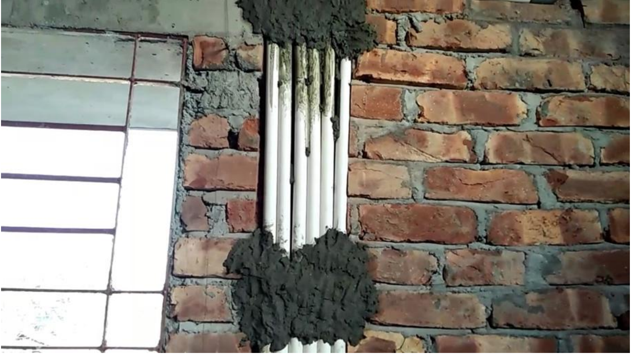
Concealed conduit and wires installation
