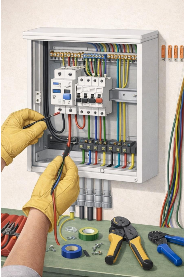
Installation & dressing of electrical distribution board
