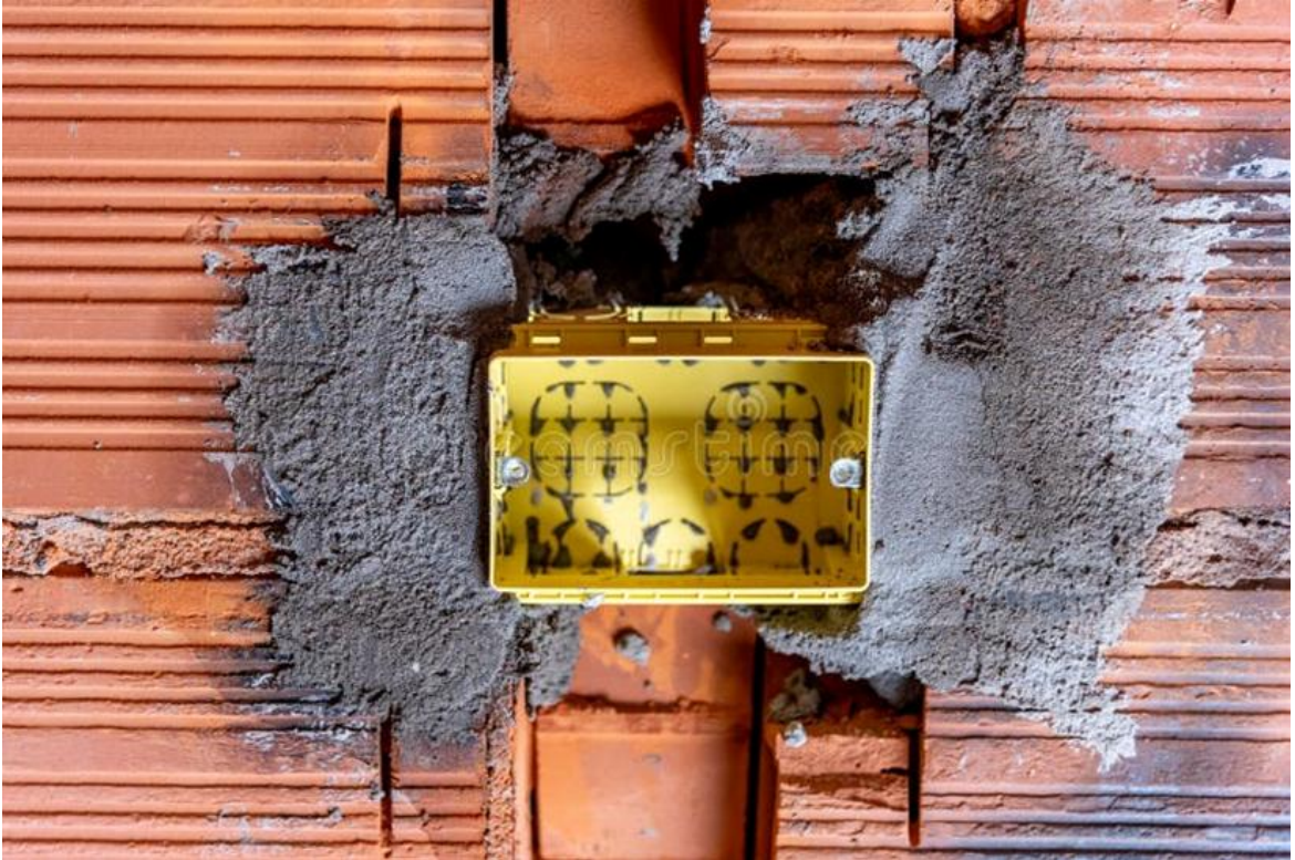
Installation of switches, sockets and fixtures into gang boxes
