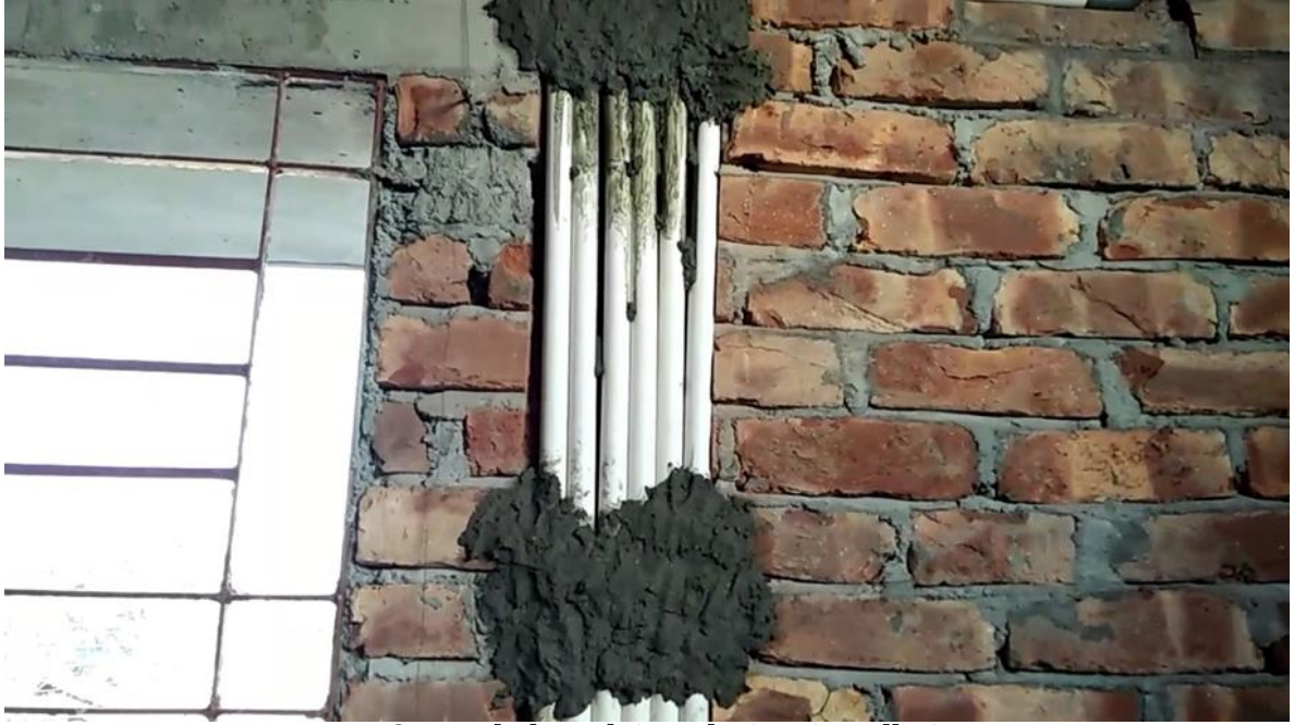
Concealed conduit and wires installation
