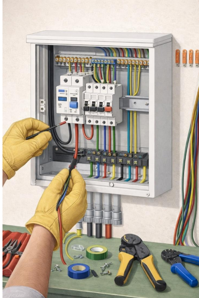
Instalation & dressing of electrical distribution board
