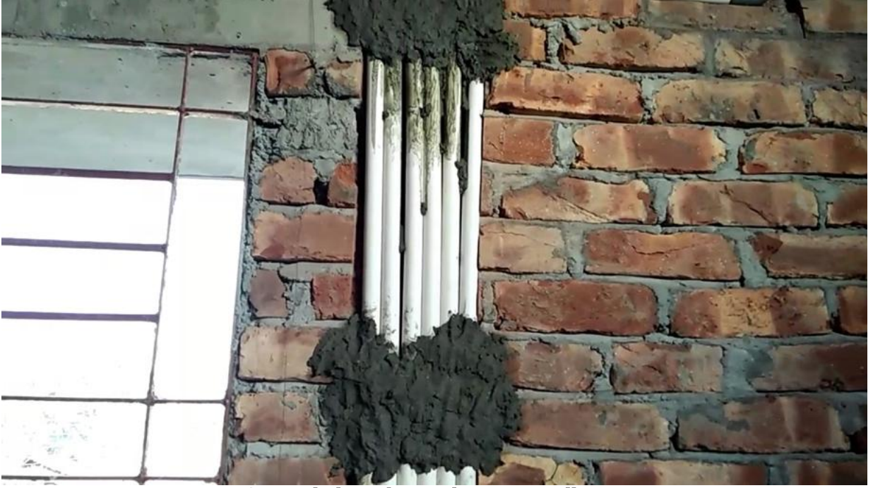
Concealed conduit and wires installation
