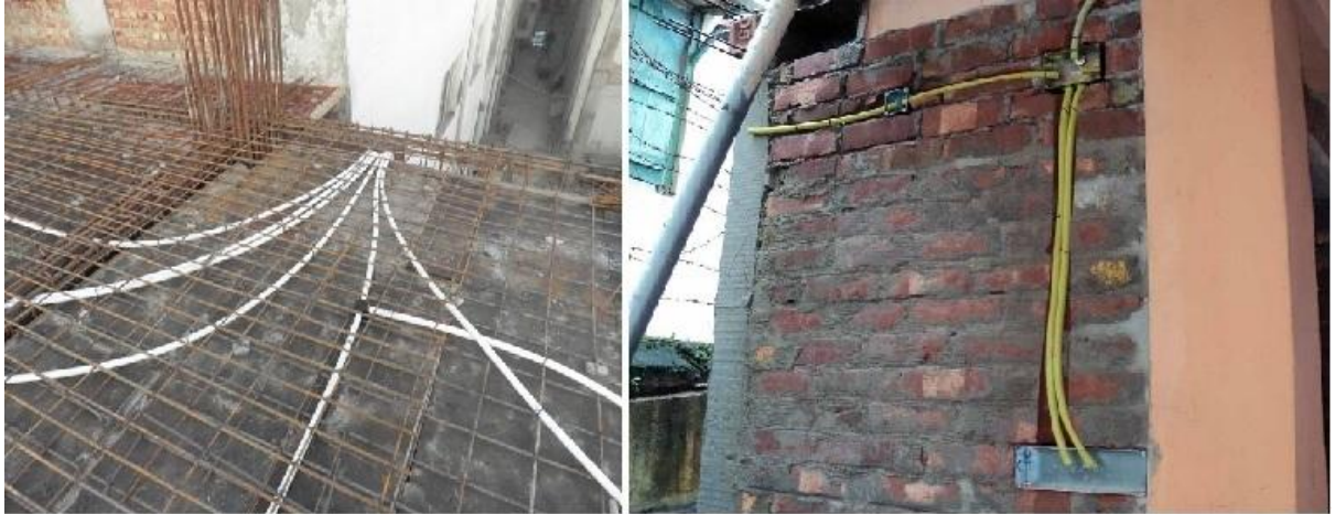
Concealed Conduit Installation in Slabs and Walls
