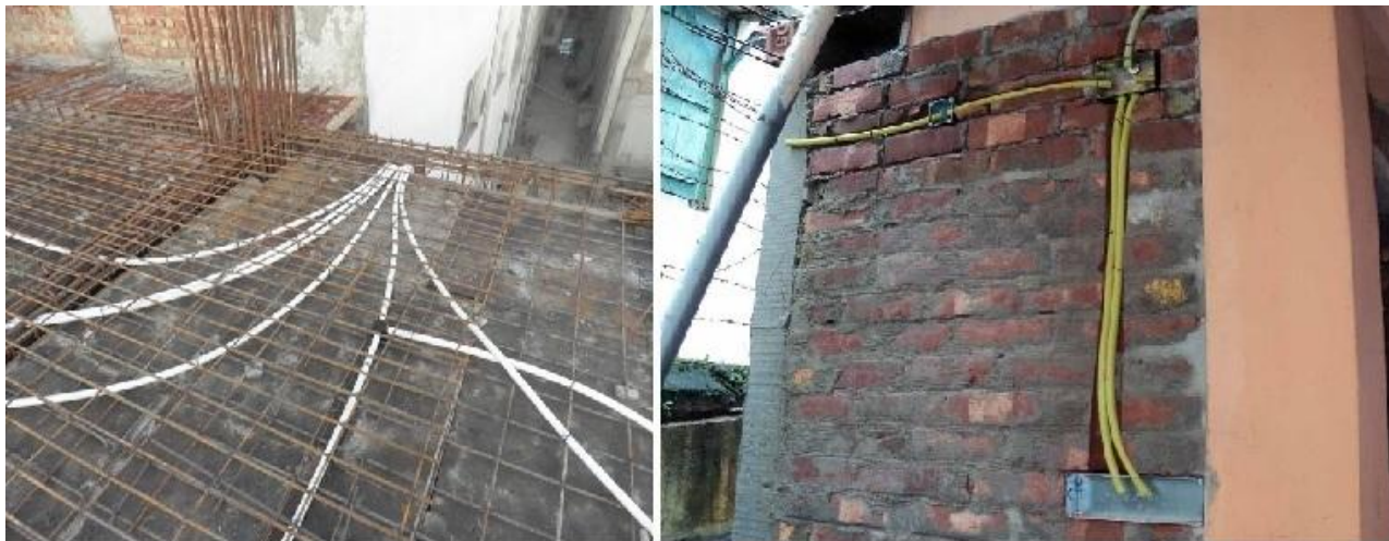
Concealed Conduit Installation in Slabs and Walls
