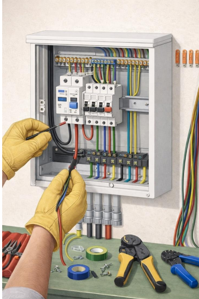
Instalation & dressing of electrical distribution board
