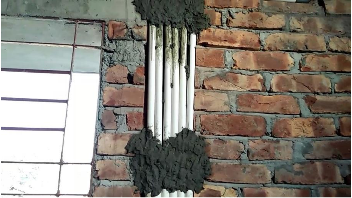
Concealed conduit and wires installation
