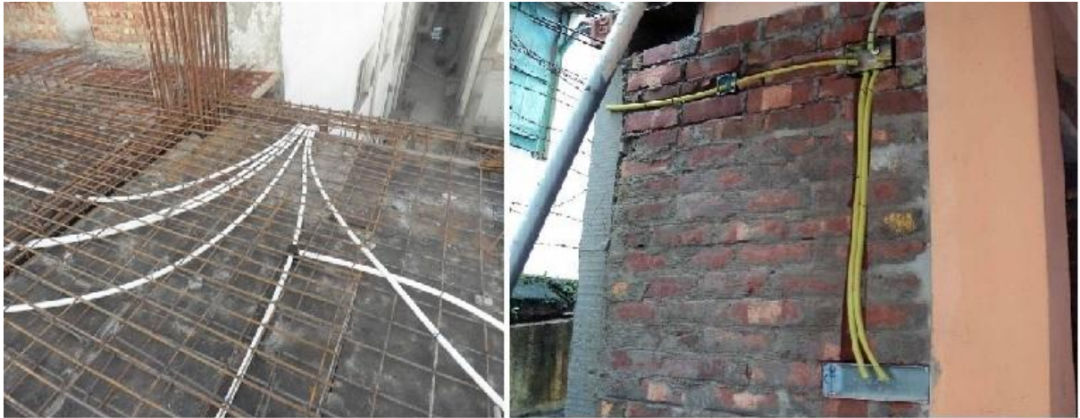
Concealed Conduit Installation in Slabs and Walls
