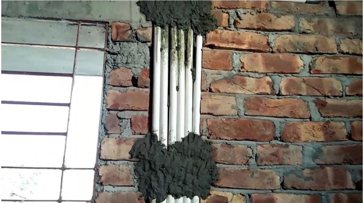
Concealed conduit and wires installation
