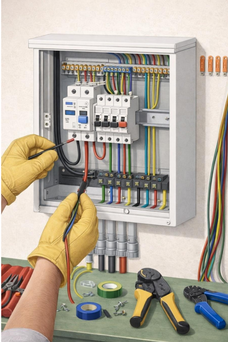
Installation & dressing of electrical distribution board
